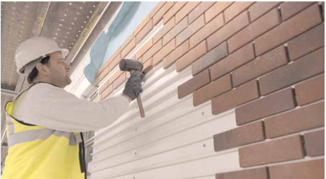
Illustrating how tiles are placed quickly and accurately prior to pointing
